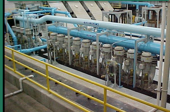
Wet Sump Installation
